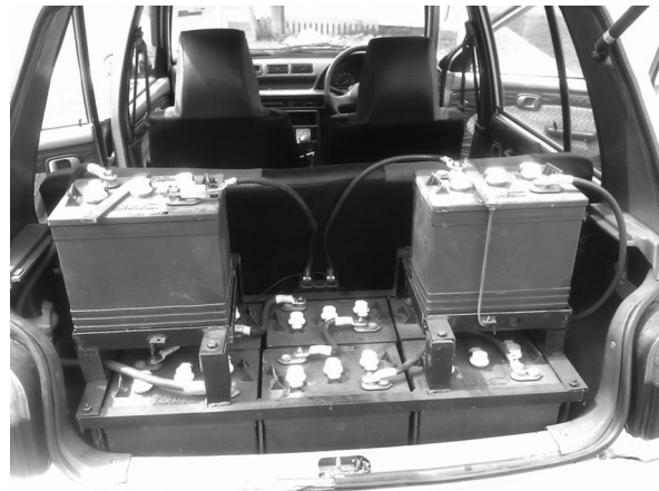
Fig. 2 8 x (6 V 225 Ah) T105 Deep cycle Lead Acid Batteries installed
