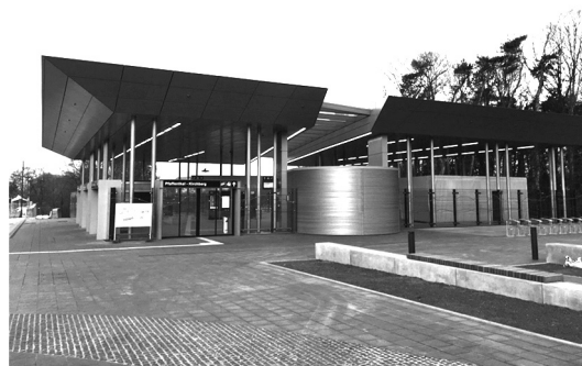
Figure 7: Funicular station (Tram side)
