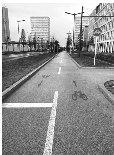
Figure 12: A newly constructed cycle path
