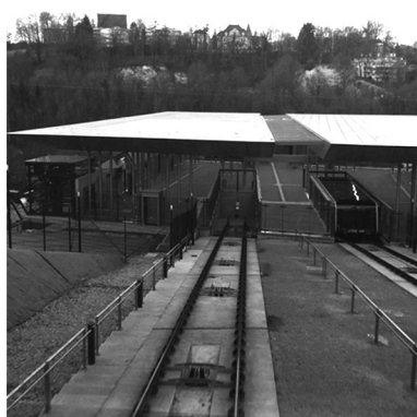
Figure 10: Funicular station (Train side)
