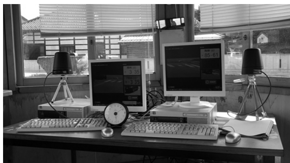
Figure 2: Installed license number authentication system
