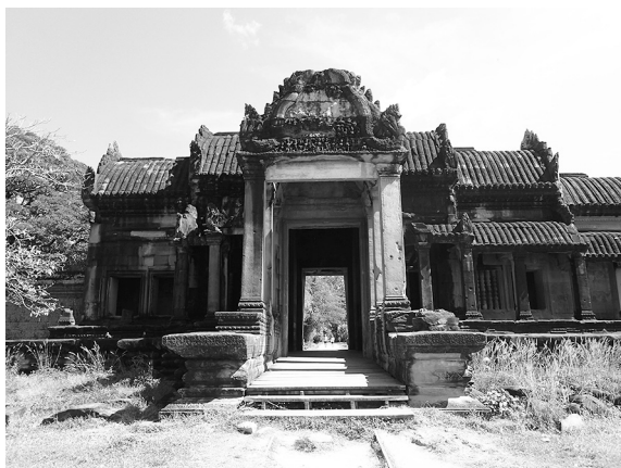
Figure 4: The west tower gate (Point (6))
