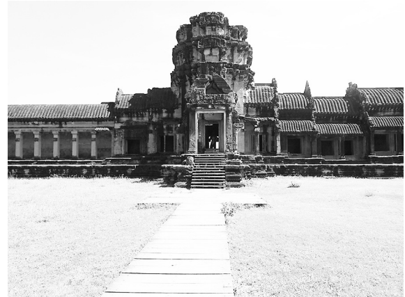
Figure 3: The west tower gate (Point (4))
