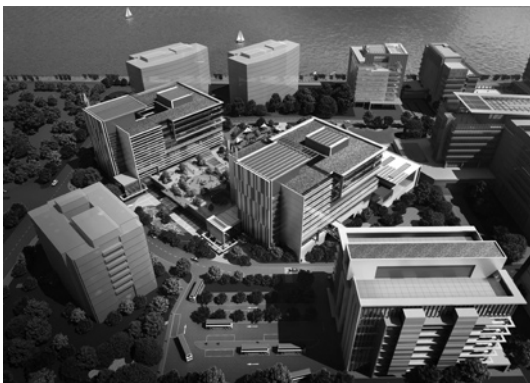
Figure 9: Hong Kong Science Park Phase 3
